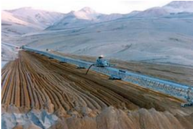
Figure 3: Dry-Stacked, Filtered Tailings Transported by Conveyor and Compacted by Dozer (Australian Government, 2016)
